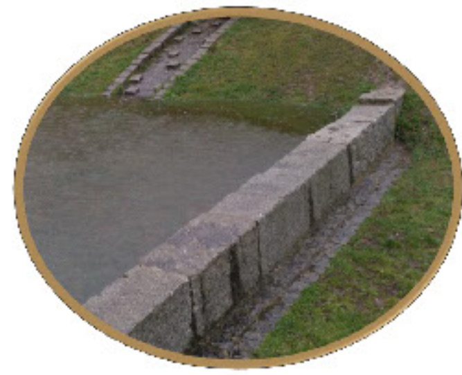
Stormwater infiltration facility
