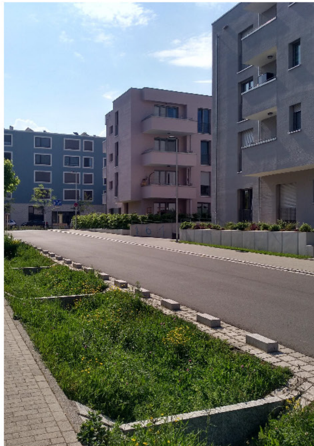
Stormwater infiltration facility
